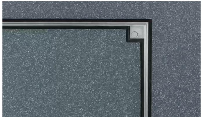
**Step 9:** Refit the cover and check there is an even gap between the cover and frame. Insert all locking screws and hand tighten to securely lock the cover. Refit all locking screw dust caps. Once the materials have fully cured, the access cover is now ready for use and service loads. Retain all spare parts, the installation and maintenance booklet and lifting/locking keys for future use.
