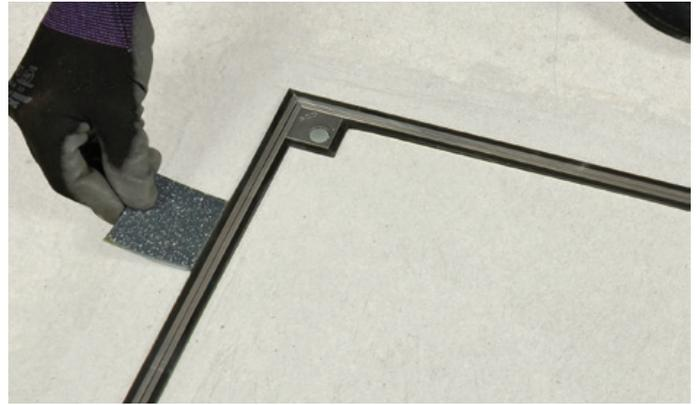
**Step 7:** Allow the concrete to sufficiently harden and dry out. Remove tape protection. The cover can now be opened with the lifting/locking keys provided. Point any gaps in the bedding under the frame if required. Refit the cover. The vinyl floor finish can now be fitted and welded to the PVC trim attached to the frame and cover as per the manufacturer's instructions.
