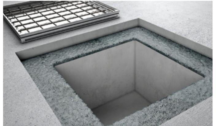
**Step 4:** Lay a mortar bed of minimum 40mm thickness all around the shaft opening the full width of the frame.
