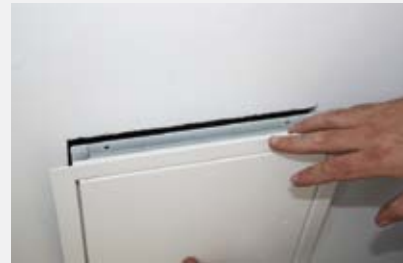
3: Take care to ensure the panel fits in to the hole
