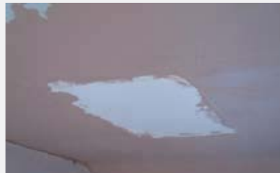
6: Finished first coat
