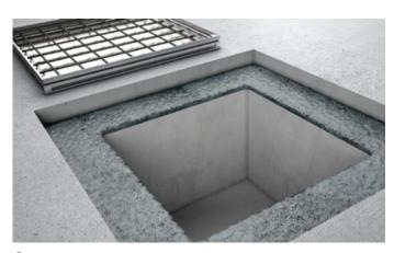
**Step 4:** Lay a mortar bed of minimum 40mm thickness all around the shaft opening the full width of the frame.
