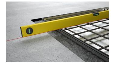
**Step 5:** Bed and level to the access cover and frame centrally over the shaft opening ensuring the top edges of the access cover and frame are at the finished vinyl floor level. When tapping down to level use a piece of wood to protect the upper surfaces. Ensure the frame is fully supported by the mortar with no voids. Allow mortar to sufficiently harden.
