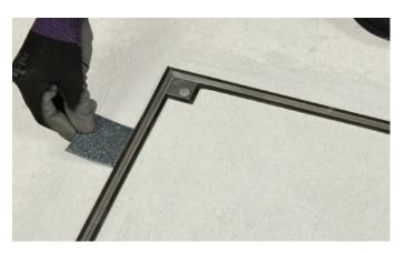
**Step 7:** Allow the concrete to sufficiently harden and dry out. Remove tape protection. The cover can now be opened with the lifting/locking keys provided. Point any gaps in the bedding under the frame if required. Refit the cover. The vinyl floor finish can now be fitted and welded to the PVC trim attached to the frame and cover as per the manufacturer's instructions.
