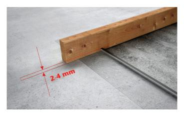
**Step 6:** Ensure the reinforcement provided is placed at the bottom of the cover. Haunch the frame fully with concrete (min 150mm wide) and fully fill the cover to within 2-4mm of its upper surface to suit the thickness of vinyl flooring to be installed. Vibrate concrete where necessary to ensure no voids and the weldable PVC trim is fully supported.
