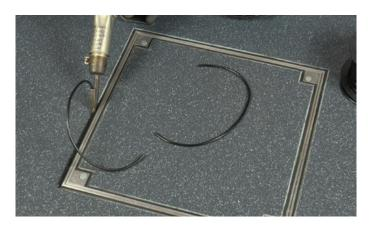
**Step 8:** Once the final floor has been fully installed, remove any excess adhesive or grout from around the cover and frame. Open the cover with the lifting/locking keys provided. Clean all surfaces and ensure the sealing areas of the cover and rubber seals are free from debris. Lubricate all seals with a suitable silicone grease.
