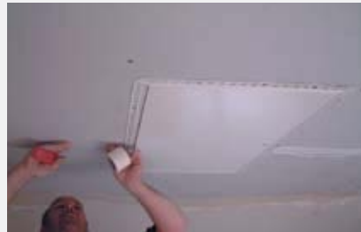
4: Tape the ceiling
