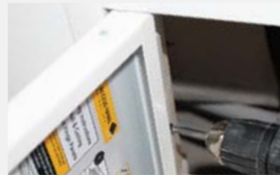
5: Hold the panel in place and use the pre-punched fixing holes on the side of the frame to secure
