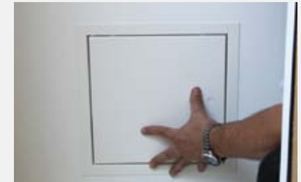
4: Ensure the picture frame sits flush with the wall or ceiling
