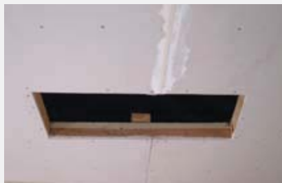
1: Cut the plasterboard to the aperture
