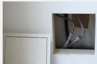
1: Prepare the hole in the wall or ceiling
